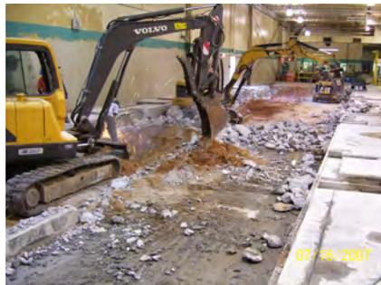
Soil removal began in July 2007 in an area approximately 20 feet by 15 feet. Based on TCLP results, it was decided that the concrete could be re-cycled. The vertical extent of the soil removal was guided by additional soil sampling, including samples collected using geoprobe equipment. Rapid turnaround from the Rogers & Callcott laboratory resulted in no delays during soil removal. Based on the geoprobe sample results, it was decided to remove soil down to the water table within the target area.
